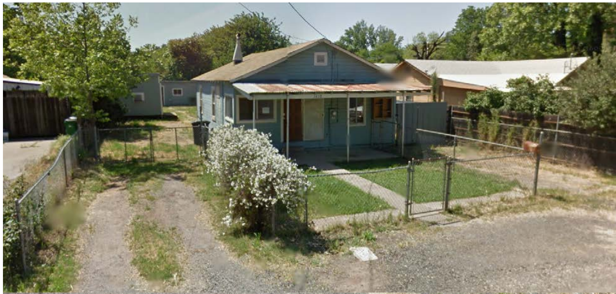
Project Site – 1438 Fetter Street
