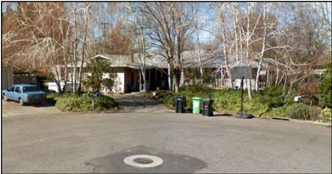
Project Site – 18 Mayfair Drive (Photo – Google Maps)
