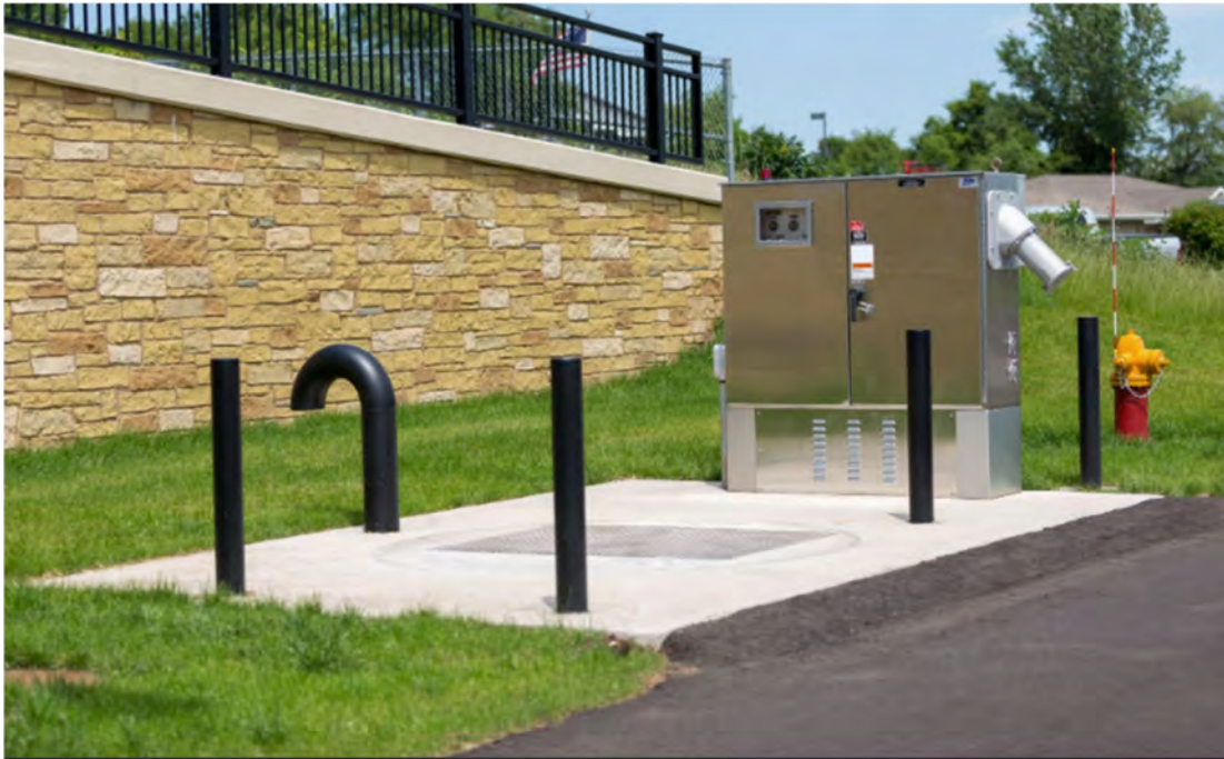
Figure 2-9. Example Transition Chamber with Vehicular Bollard Protection
