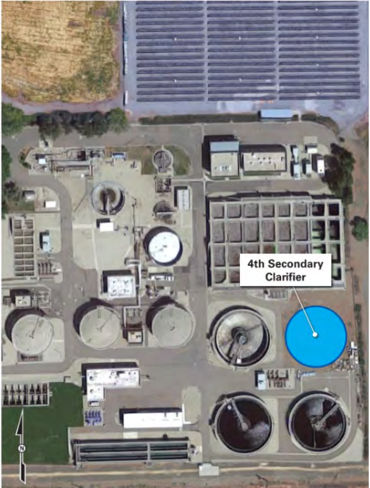
Figure 4.2 Fourth Secondary Clarifier
