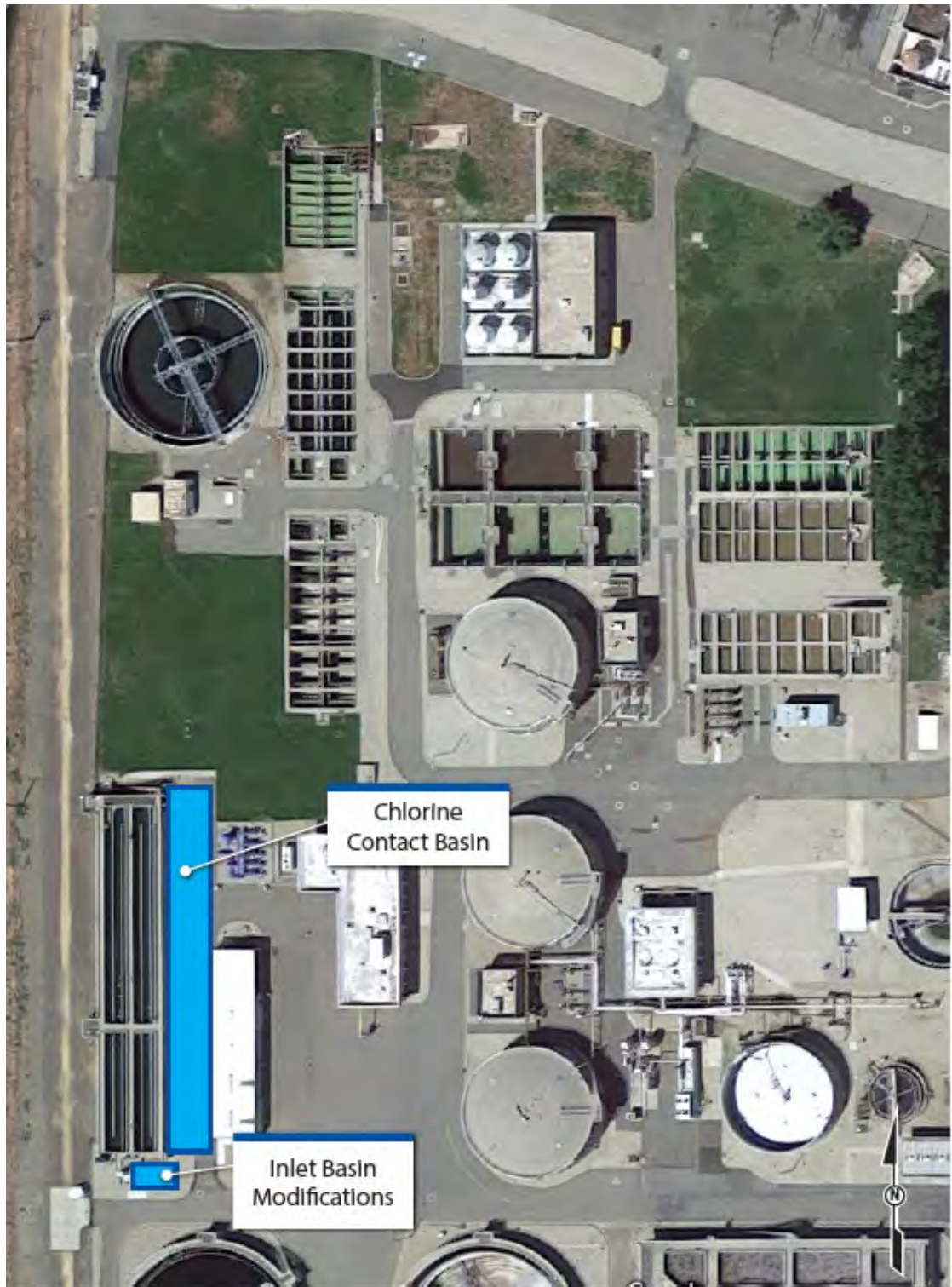
Figure 4.6 Chlorine Contact Basin
