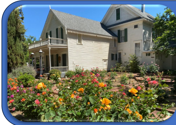
C.F. Lott Home. A Victorian revival style structure, the C.F. Lott Home was built in 1856 by “Judge” Lott, a gold-rush pioneer who helped form California’s government. Sank Park encompasses the entire city block that Judge Lott bought in 1855 for $200. The garden contains a profusion of flowers, including an outstanding hybrid rose area.
