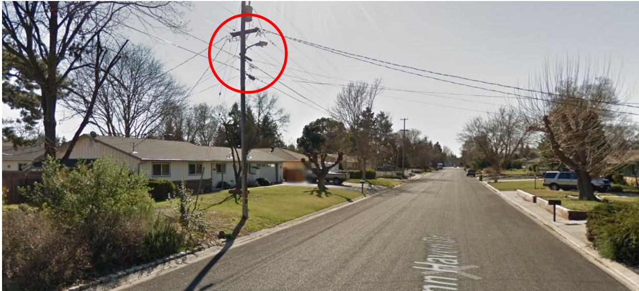
Pole Mounted Light Fixture – Google Maps
